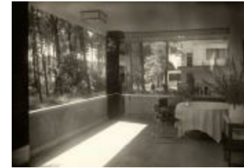
Masters' House Interior (2019.3.8)
