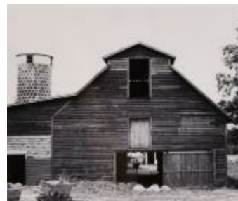
Barn and Silo with Cow in Doorway (2016.24.3)
