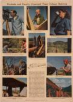
"Students and Faculty Construct their College Building" (1995.8.1)
