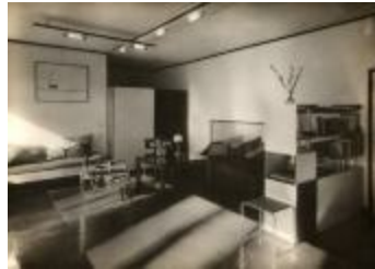
Masters' House Interior (2019.3.7)
