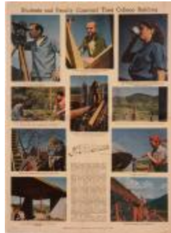
"Students and Faculty Construct their College Building" (1995.8.1)
