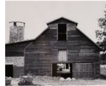
Barn and Silo with Cow in Doorway (2016.24.3)
