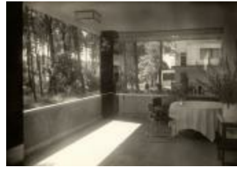
Masters' House Interior (2019.3.8)
