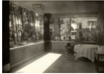
Masters' House Interior (2019.3.8)
