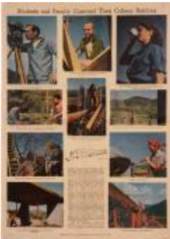
"Students and Faculty Construct their College Building" (1995.8.1)
