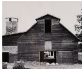
Barn and Silo with Cow in Doorway (2016.24.3)
