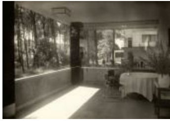
Masters' House Interior (2019.3.8)
