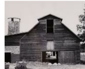
Barn and Silo with Cow in Doorway (2016.24.3)
