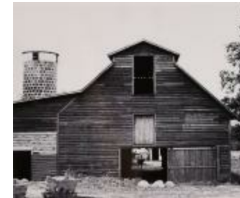
Barn and Silo with Cow in Doorway (2016.24.3)
