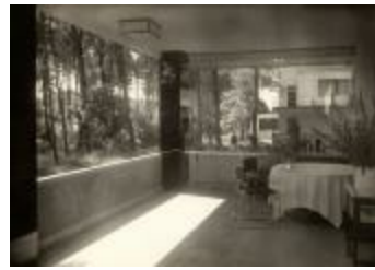
Masters' House Interior (2019.3.8)
