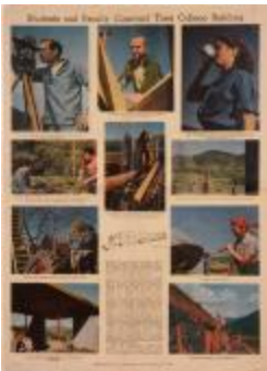
"Students and Faculty Construct their College Building" (1995.8.1)
