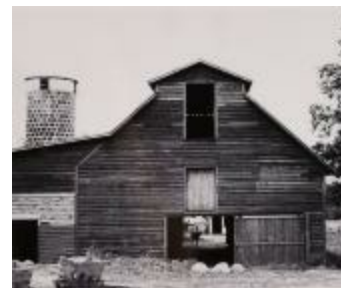
Barn and Silo with Cow in Doorway (2016.24.3)
