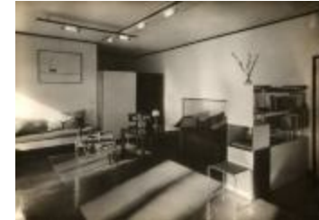
Masters' House Interior (2019.3.7)
