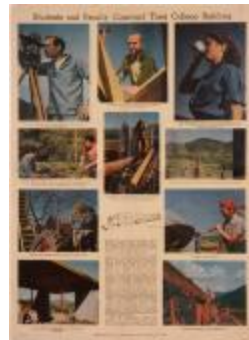
"Students and Faculty Construct their College Building" (1995.8.1)
