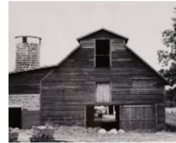
Barn and Silo with Cow in Doorway (2016.24.3)
