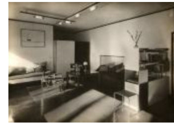
Masters' House Interior (2019.3.7)
