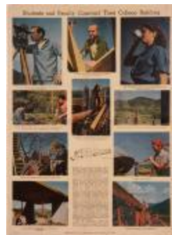
"Students and Faculty Construct their College Building" (1995.8.1)
