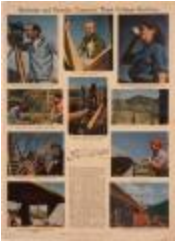
"Students and Faculty Construct their College Building" (1995.8.1)
