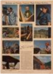
"Students and Faculty Construct their College Building" (1995.8.1)
