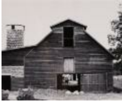
Barn and Silo with Cow in Doorway (2016.24.3)
