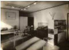
Masters' House Interior (2019.3.7)
