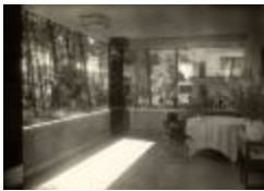
Masters' House Interior (2019.3.8)
