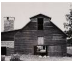
Barn and Silo with Cow in Doorway (2016.24.3)
