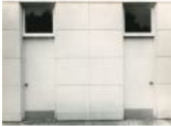
New Amoco Station, North Carolina (1995.14.8)
