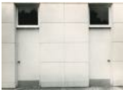
New Amoco Station, North Carolina (1995.14.8)
