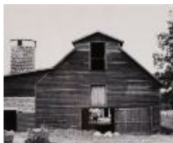
Barn and Silo with Cow in Doorway (2016.24.3)
