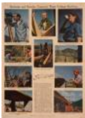
"Students and Faculty Construct their College Building" (1995.8.1)
