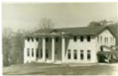
Blue Ridge Assembly Building (2003.7.1.08)
