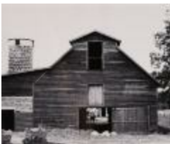
Barn and Silo with Cow in Doorway (2016.24.3)
