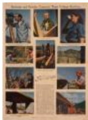
"Students and Faculty Construct their College Building" (1995.8.1)
