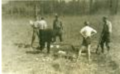
Black Mountain College Work Program at Blue Ridge Assembly (2003.7.1.22)
