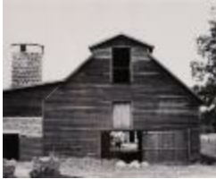
Barn and Silo with Cow in Doorway (2016.24.3)
