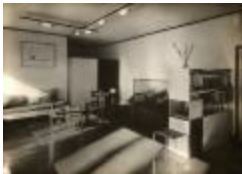
Masters' House Interior (2019.3.7)
