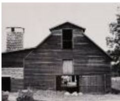
Barn and Silo with Cow in Doorway (2016.24.3)
