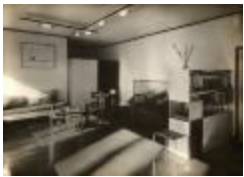
Masters' House Interior (2019.3.7)
