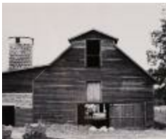
Barn and Silo with Cow in Doorway (2016.24.3)
