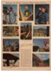
“Students and Faculty Construct their College Building” (1995.8.1)
