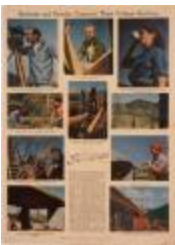
"Students and Faculty Construct their College Building" (1995.8.1)
