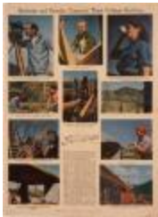
"Students and Faculty Construct their College Building" (1995.8.1)
